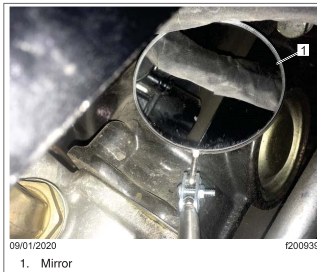
Fig. 3, Inspection by Mirror
