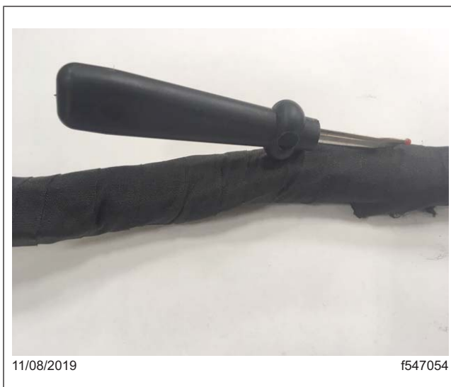
Fig. 4, Cutting an Opening into the Fiber Wrap
