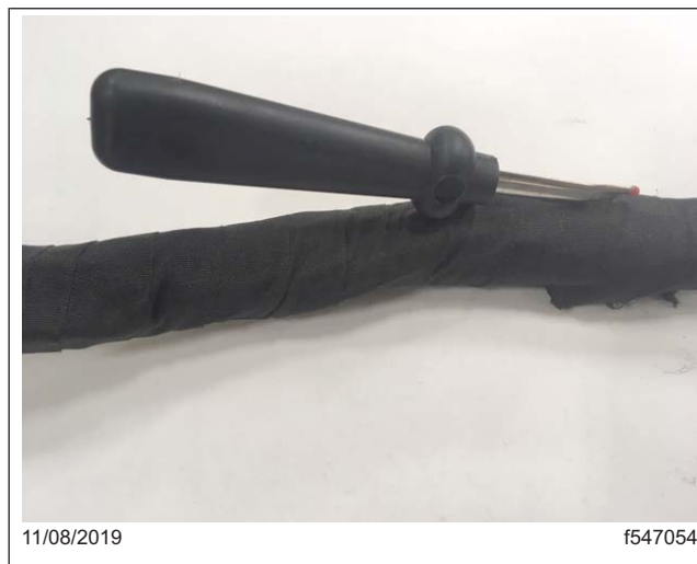
Fig. 3, Cutting an Opening into the Fiber Wrap
