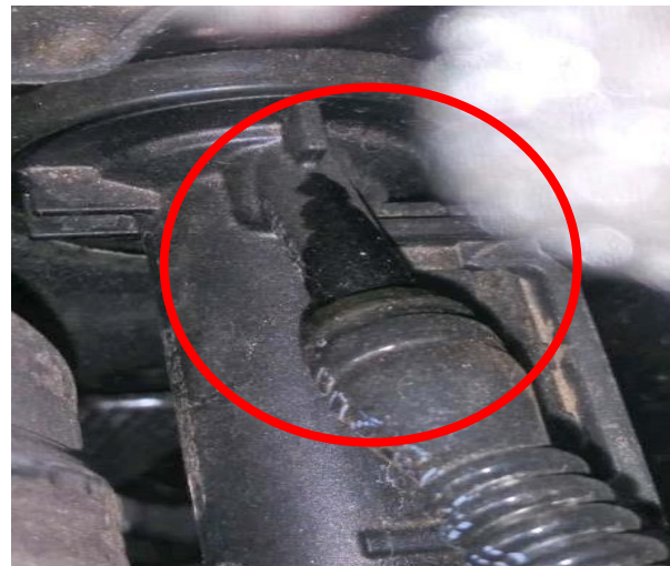
SAMPLE of Leak/Seepage
