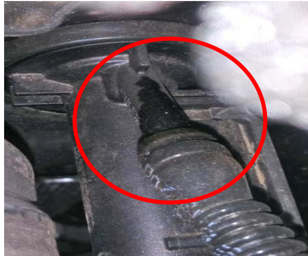
SAMPLE of Leak/Seepage
