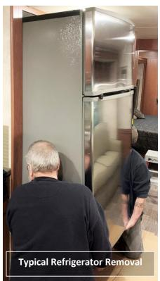
Be aware of the potential for damage to the refrigerator cabinet face frame and use safeguards to prevent damage from happening.
