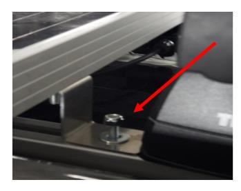
10. Insert bolt through the front leg of the solar panel. Install the washer and locking nut. Tighten with an 11mm nut socket.
