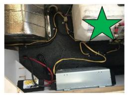
This is correct, the inverter is installed on the panel and the fuse holder is installed on the panel and has the plastic cover installed.
