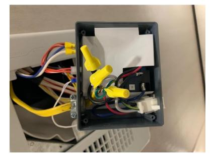
9. Once all the old connections have been replaced with the proper yellow wire nuts, wrap the individual connections in electrical tape.
