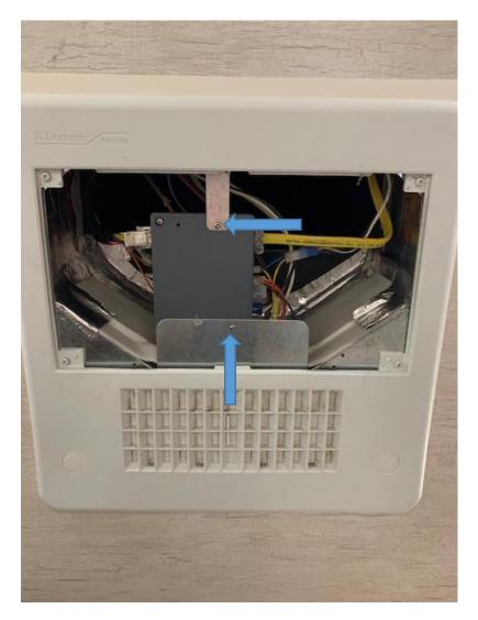
4. Lower the electrical box down so that all four screws on the electrical box are exposed.
