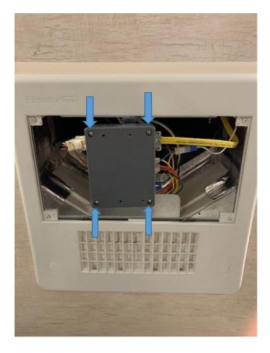
5. Remove all four screws holding the electrical cover in place and then remove the cover.
