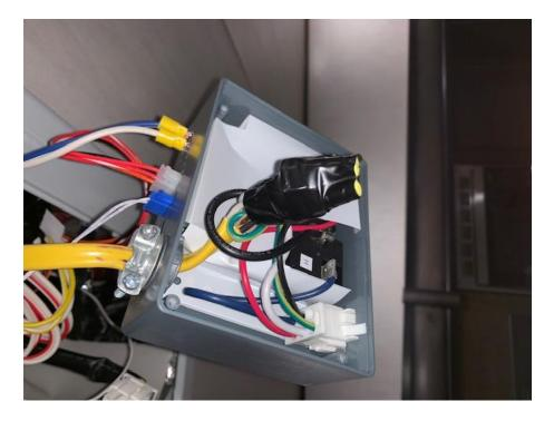
10. Once each connection is wrapped individually in electrical tape, wrap all three connections together with an additional piece of electrical tape.
