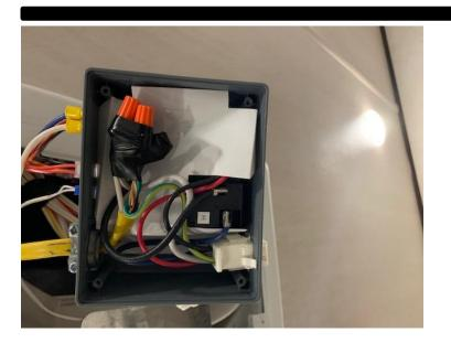
6. Pull the wires out of the box and separate them so that each connection is clearly visible. Remove electrical tape from each connection.
