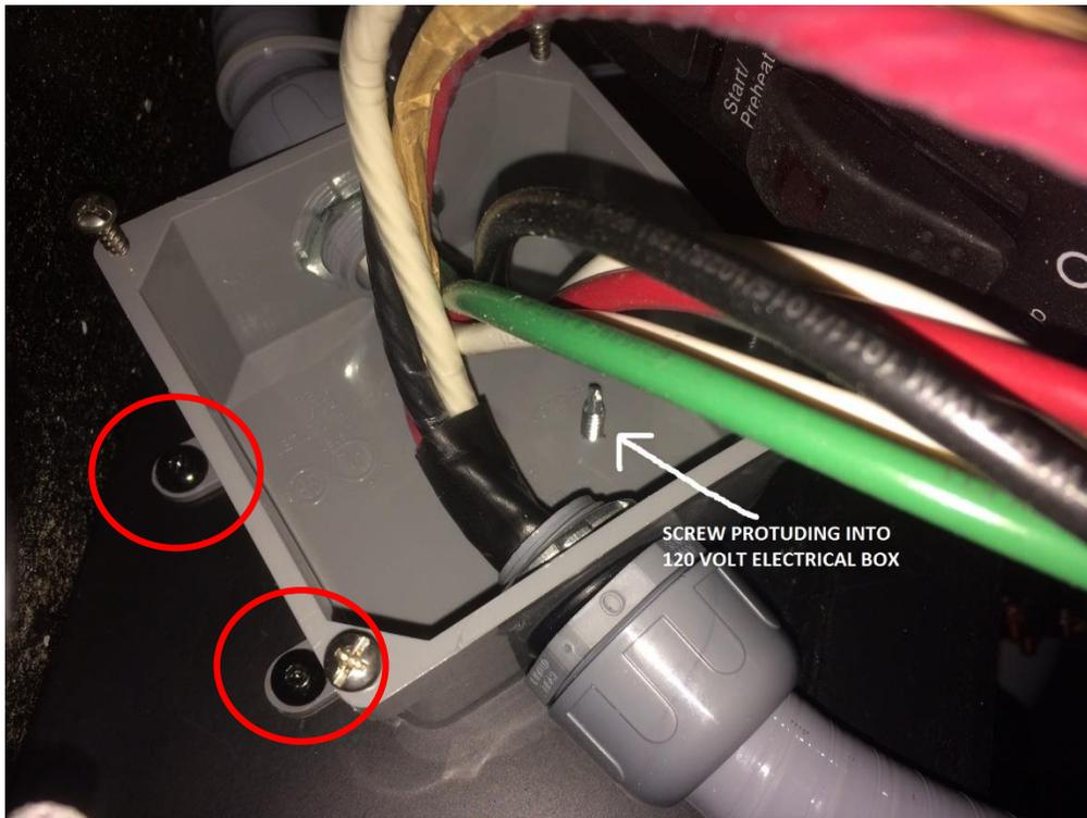
6. Caulk the hole in the junction box that was left from removing the screw to prevent any water intrusion.
