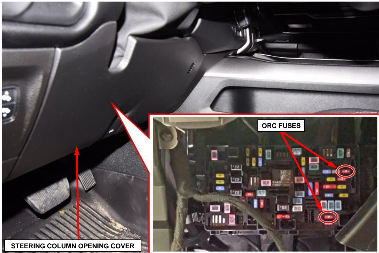
Figure 6 – ORC Fuses F28 and F65
