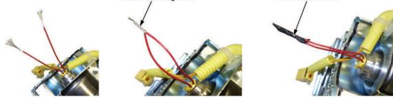
3.3. Tape the twisted ends with electrical tape.
