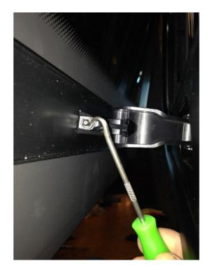
5. Remove the pin that secures the latch to the glass.
