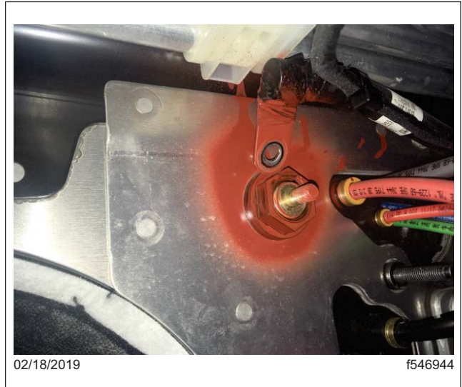
Fig. 5, GNDE Engine-Side Pass-Through Stud
