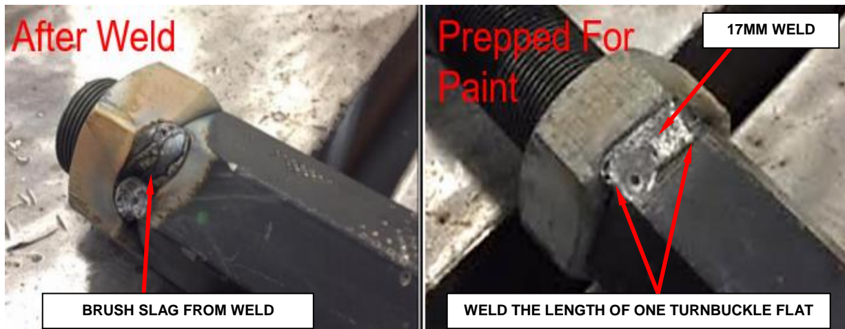
Figure 10 – Prepare areas for Paint
