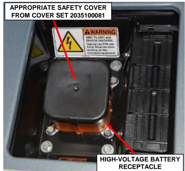
Figure 17 – High-Voltage Battery Receptacle Safety Cover
