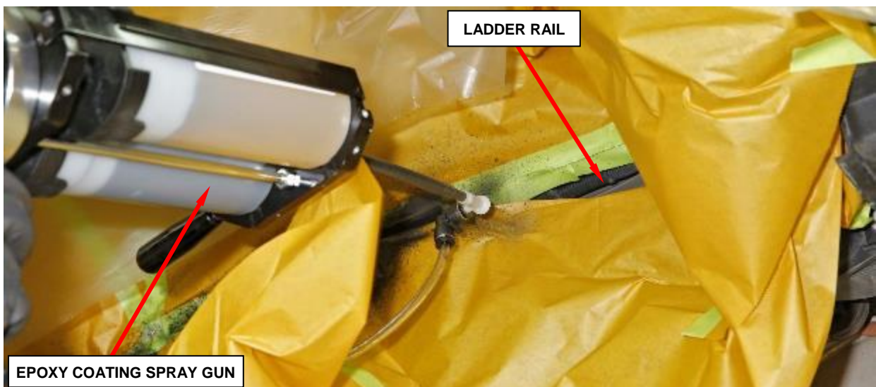
Figure 10 – Apply Epoxy Coating to Ladder Rail through Wheelhouse Opening
