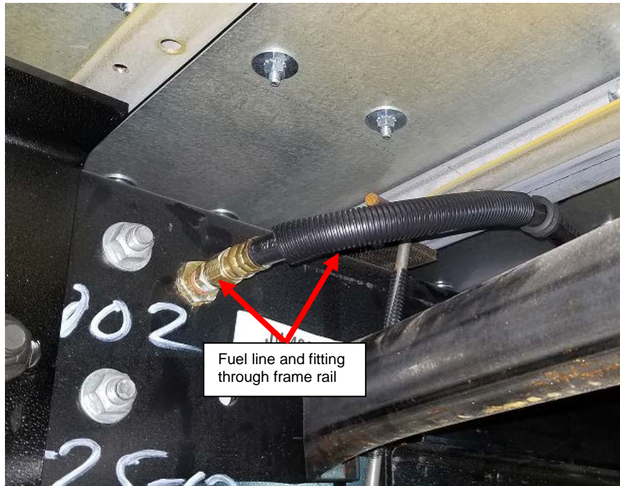
Figure 4: Installation of Fuel Line in Fitting through the Frame Rail
