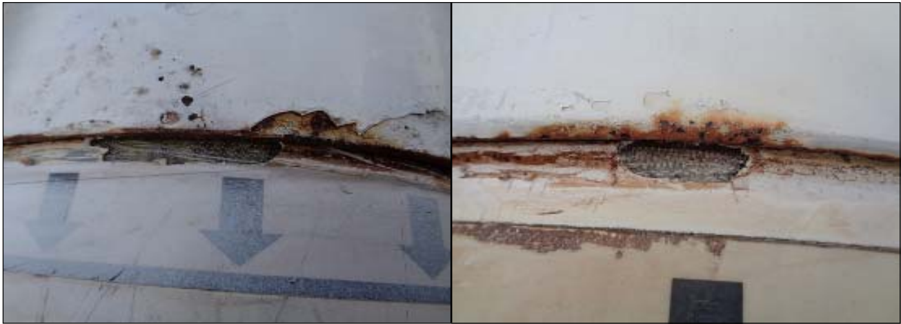
Figure 2 — Examples Of Gelcoat Damage
