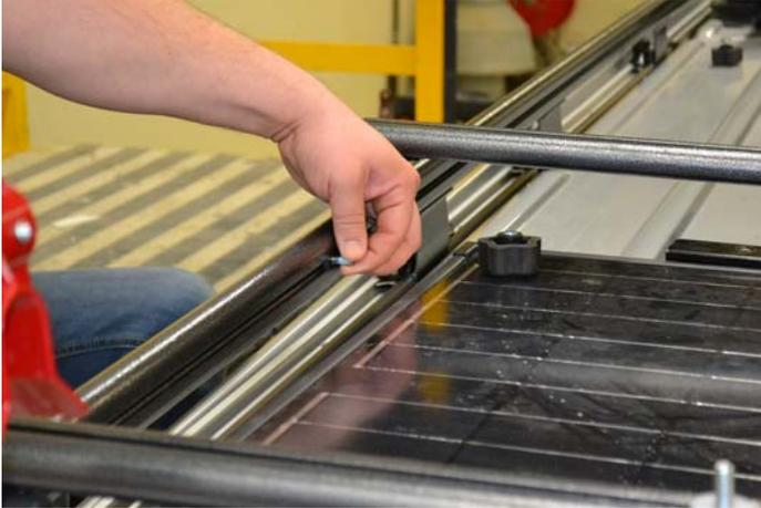
10. Install new red plastic saddles on side support rails by placing hole in saddle over T-bolt and snapping saddle over side support rail. Make sure T-bolt goes through the hole in the red saddle.
