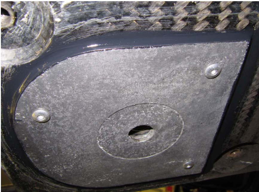
Fig 11: Detail view of the RPS Plate surrounding sealed with Scotch-Weld DP 490
