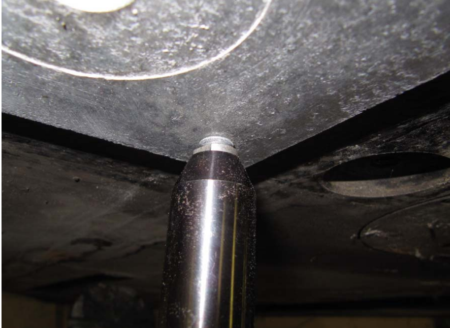
Fig 8: Installation of the blind rivet with the Avdel installation device Genesis nG3
