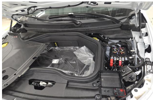
Figure 4 – KM Power Distribution Center
