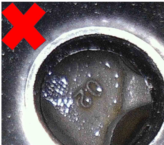
Fig. 5 Umbrella Valve Seal - Missing
