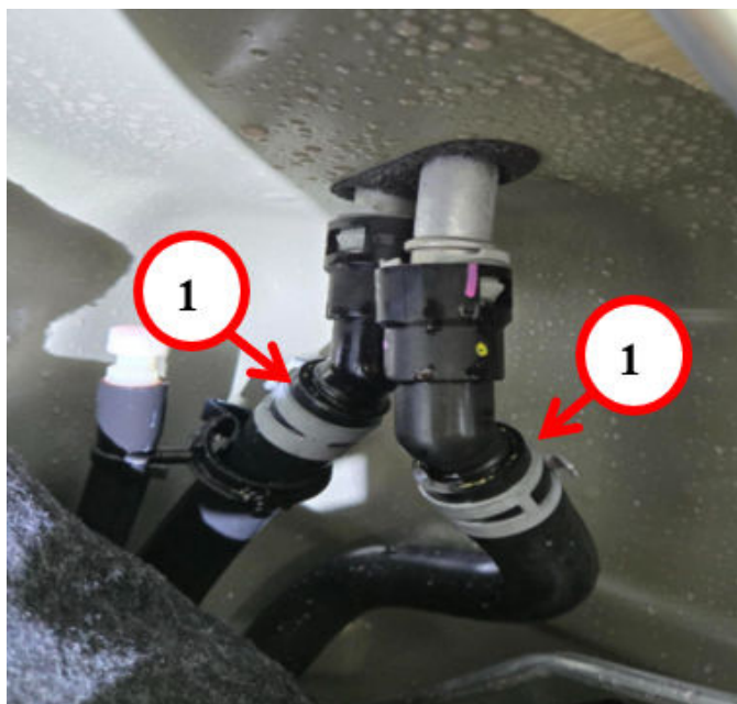
Fig. 2 Rear Coolant Hoses
