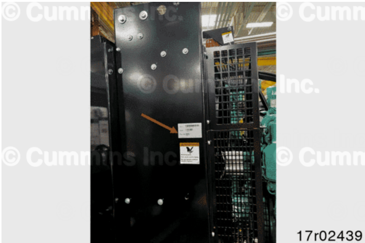
Figure 1, A068H458, A076T598, A077Y449, A079J255 and A079N739 Part Number Location
