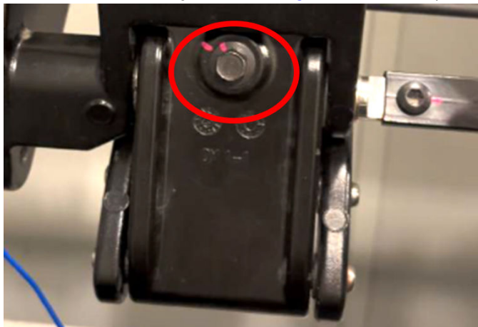
Fig. 2 Motor Shaft Joint Bolt
