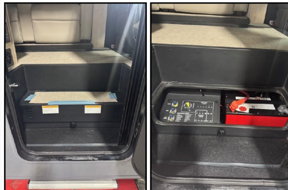
Fig. 6 — Entry step cover removed for access to the DCD panel.
