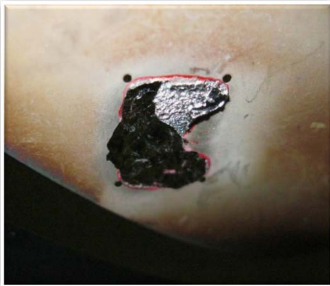
Terminal detached with removed conductor and solder Not warrantable
